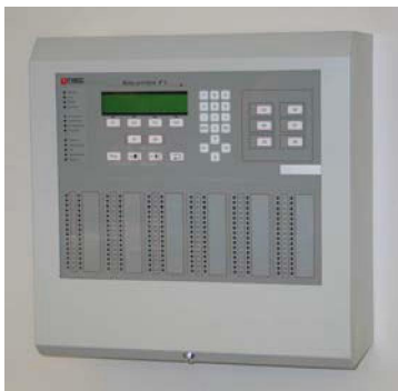
(Photo of housing B2 incl. FCP „Solution F1-18“ and zone LEDs)
