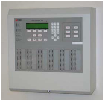
(Photo of housing A2 incl. FCP „Solution F1-6“ and zone LEDs)
